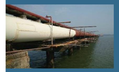
In a competitive tender situation, Kirloskar Corrocoat was awarded and successfully completed a prestigious order for Mumbai Port Trust. The contract was for the external coating of a pipeline at the Butcher Island complex and involved surface preparation and coating application both on land and over the sea.
