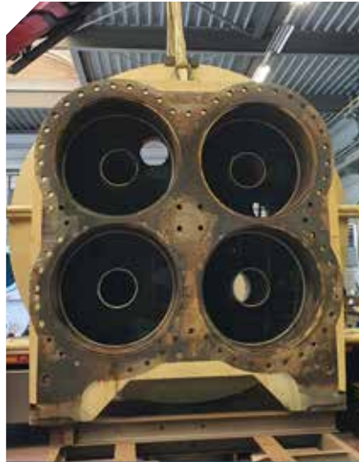
Cooling water area before protective coating
