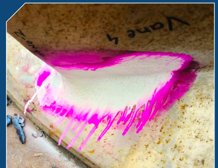
Dye Penetration Test
